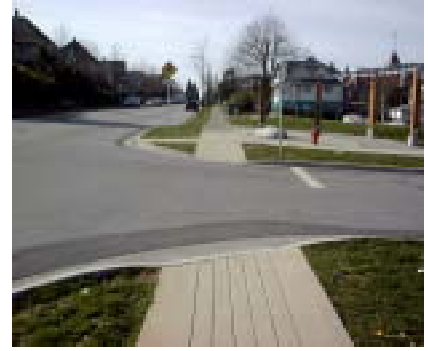
Figure 3–9: Examples of Grooves in Sidewalk
