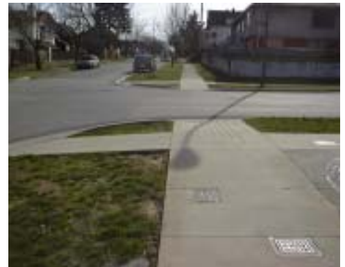
Figure 3–10: Examples of Grooves in Sidewalk
