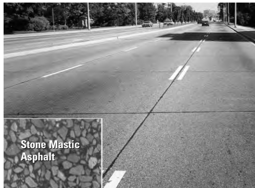
Photo 4-4: Reconstructed Municipal Road Composite Pavement with SMA Surface Course
