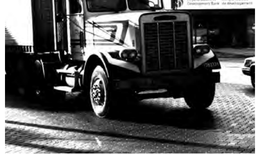
Photo 4-6: Interlocking Concrete Pavers Used to Reconstruct City Street
