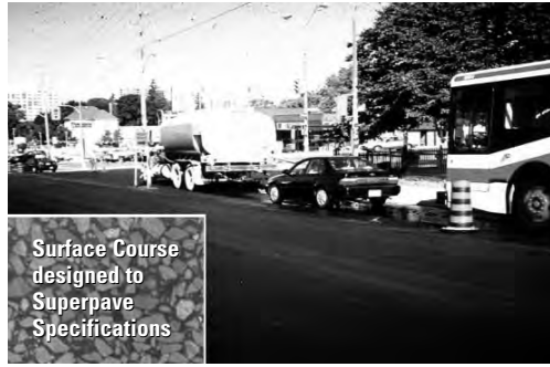
Photo 4-2: Municipal Road Composite Pavement, with Water Cooling Before Traffic Use
