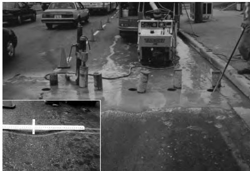
Photo 2-4: Evaluating the asphalt concrete rutting of a deep strength flexible pavement
