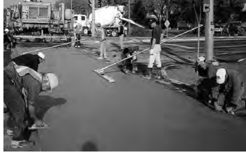
Photo 4-5: Thin Composite Whitetopping of a Municipal Connector Highway Intersection
