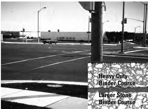
Photo 4-3: Reconstructed Municipal Road Intersection Deep Strength Flexible Pavement
