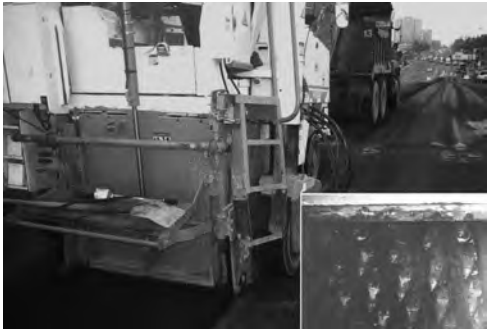
Photo 4-1: Precision Milling to Remove Asphalt Concrete Instability Rutting
