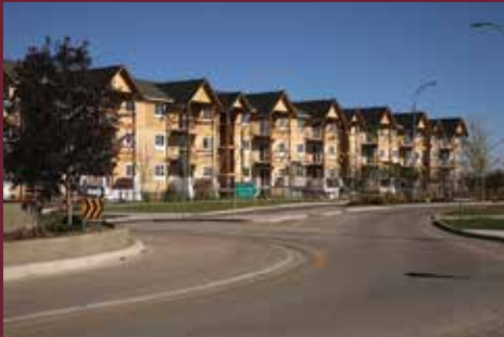
Town homes under construction in the SunRidge neighbourhood of the City of Lethbridge, AB (Credit: City of Lethbridge)
