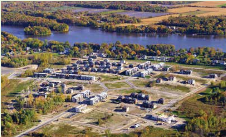
Aerial view during construction of the Urbanova neighbourhood in Ville de Terrebonne, QC (Credit: Ville de Terrebonne)
